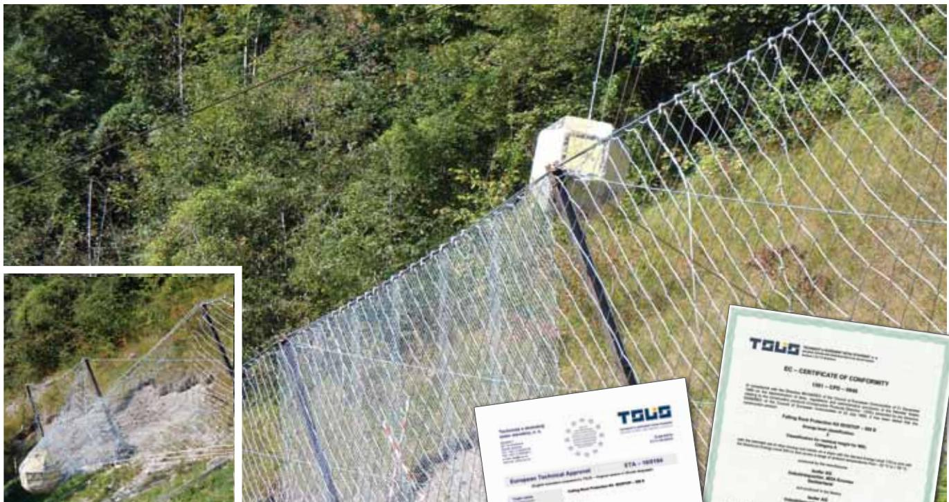
Our ISOSTOP E systems have passed the suitability test in accordance with the ETAG 027 guideline with the best possible result. After testing with 100 % nominal energy, a residual height of more than 50 % of the original height was measured in the impact zone. This corresponds to performance category A.
